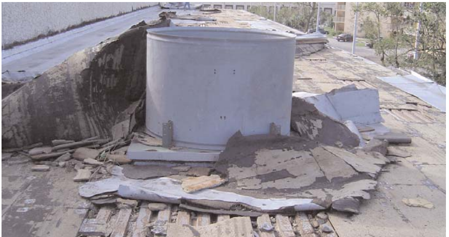
Asphalt membrane roof failed due to high winds even though fasteners remain attached.
