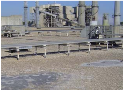
Before roofing work.
